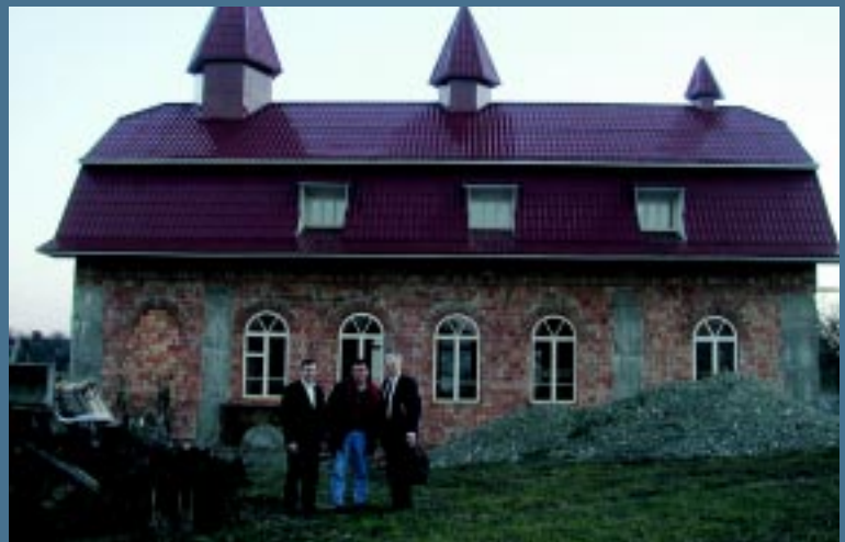
The newly constructed meeting place in Tereblecea
