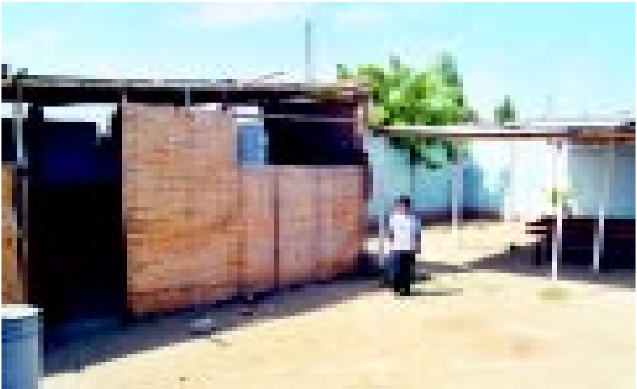
Inside the Mount Olive Baptist Church before construction began. The main auditorium was under a temporary tin roof and the Sunday School rooms (at left) were made out of straw mats.
